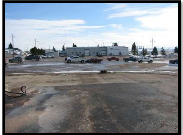
Parking, Water Dept. Looking South
