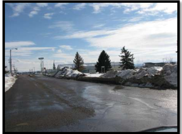
Storm Drainage to Storm Inlet
