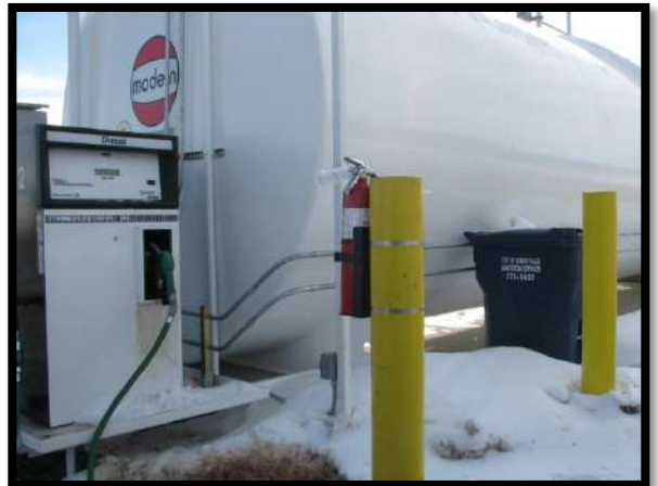
Dispenser at Fuel Station
