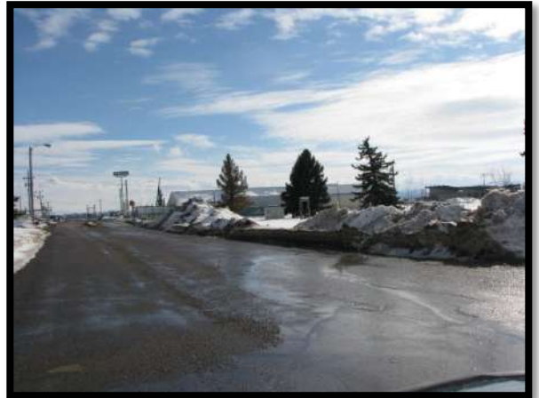
Storm Drainage to Storm Inlet
