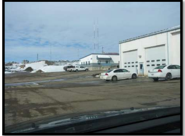
Street/Sanitation, Maintenance Shop
