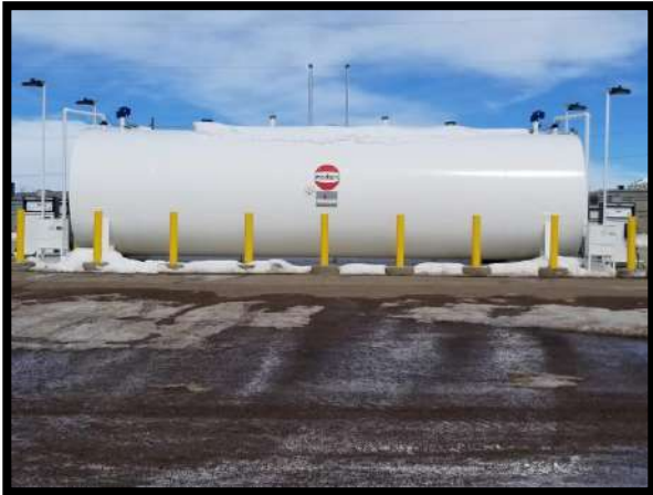
Fuel station, View Facing North
