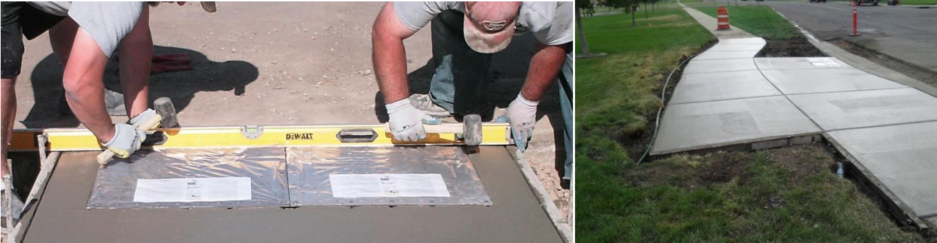
Left: Two concrete finishers place a truncated dome in concrete using a level Right: A recently finished midblock crossing with a landing
