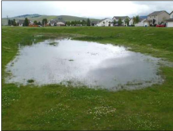
Figure 5.2-1. Infiltration Basin Source: HDR
