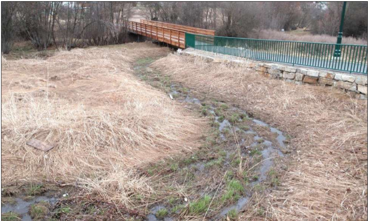
Figure 5.6-2. Meandering Biofiltration Swale
