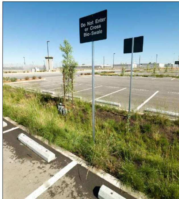
Figure 5.6-5. Biofiltration Swale Sign
