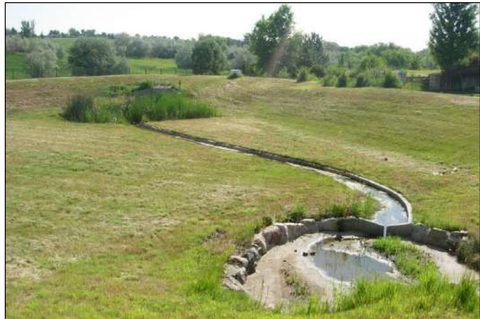
Figure 5.7-3. Pretreatment Forebay and Trickle Channel Source: Courtesy of UDFCD
