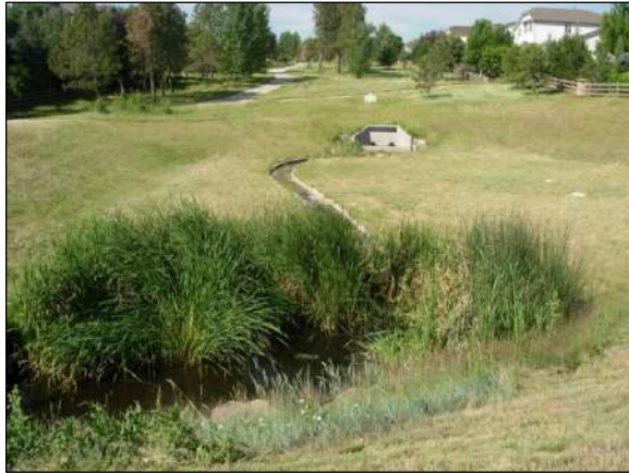
Figure 5.7-1. Extended Detention Basin Source: Courtesy of UDFCD
