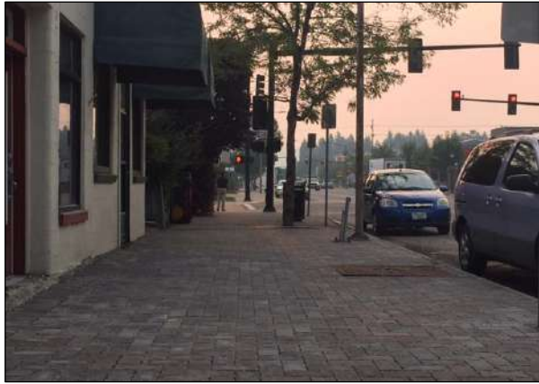
Figure 5.4-1. Permeable Interlocking Concrete Pavers in Bozeman
