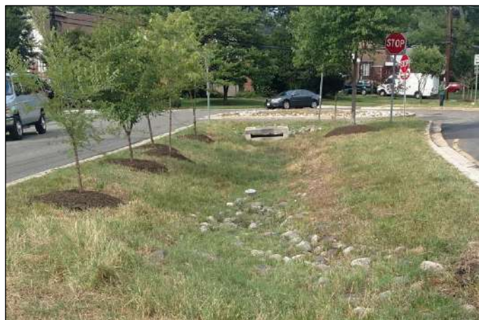
Figure 5.2-2. Infiltration Basin with Outlet Structure
