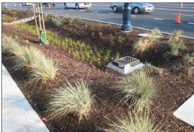
Figure 5.3-5. Online Bioretention Area with Overflow Outlet Structure
