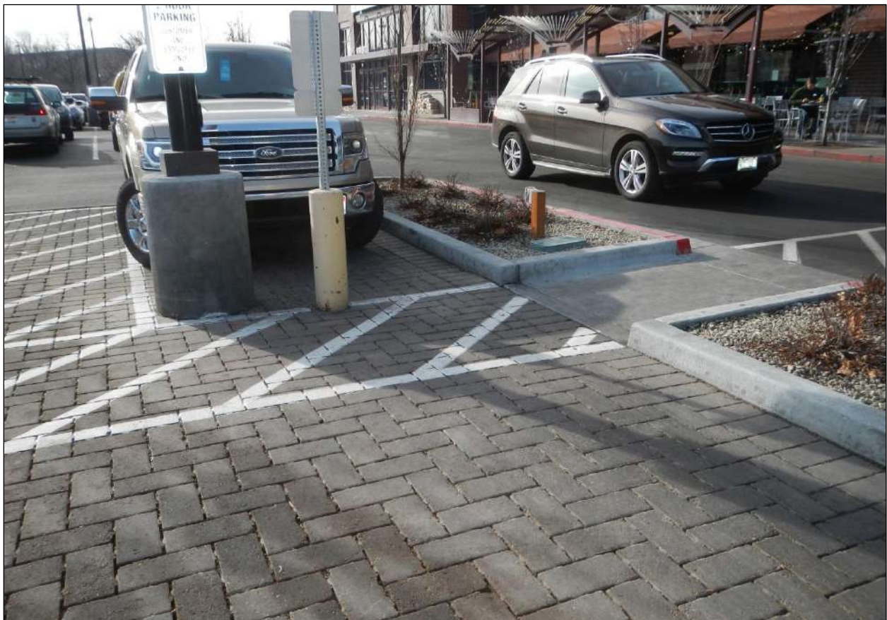
Figure 5.4-2. PICP Parking Lot Application
