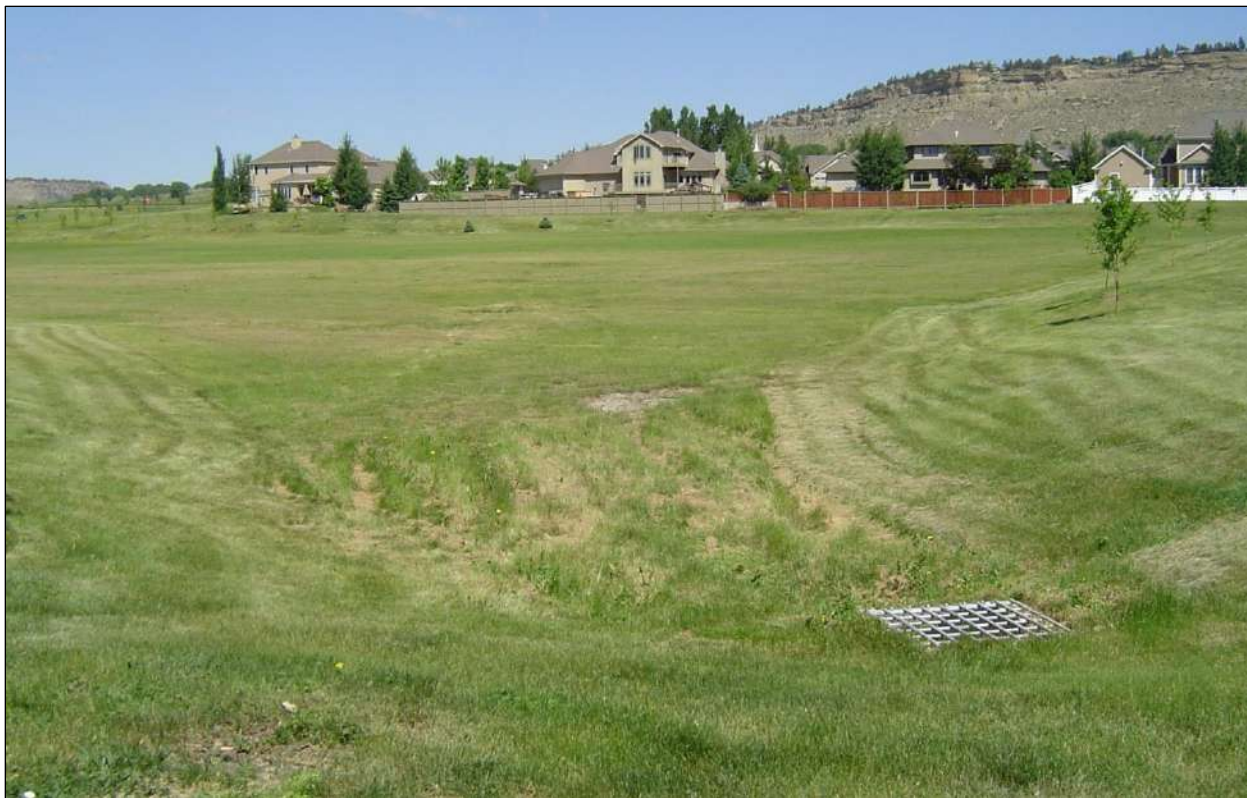
Figure 5.7-2. Detention Basin in Billings, Montana
