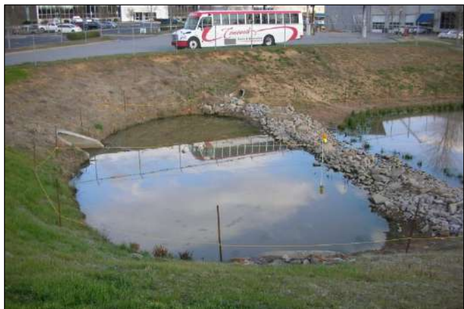
Figure 5.8-3. WDB Pretreatment Forebay
