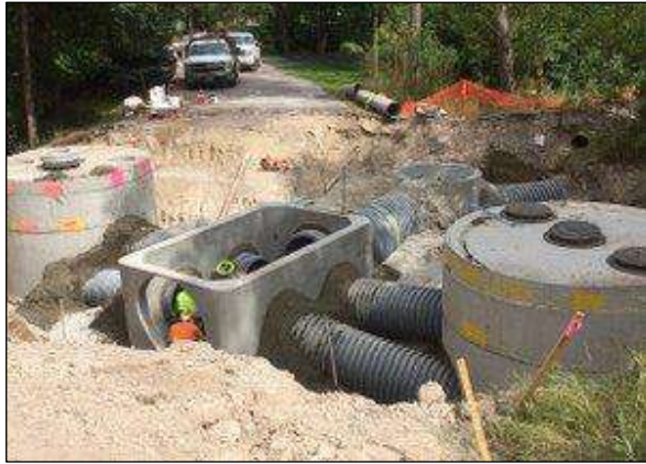
Figure 5.9-1. Proprietary Treatment Device Installation
