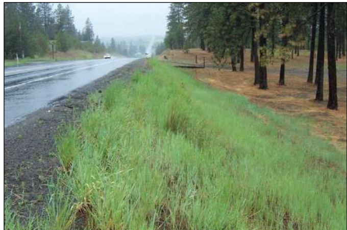
Figure 5.5-2. Dispersion Area Adjacent to a Roadway
