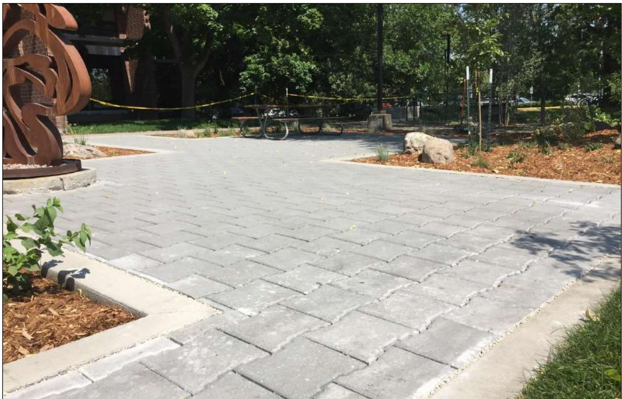
Figure 2-5. Permeable Interlocking Concrete Pavers Walkway Application
