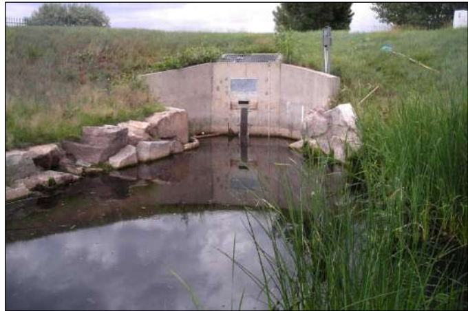
Figure 5.7-4. Micropool and Outlet Structure
