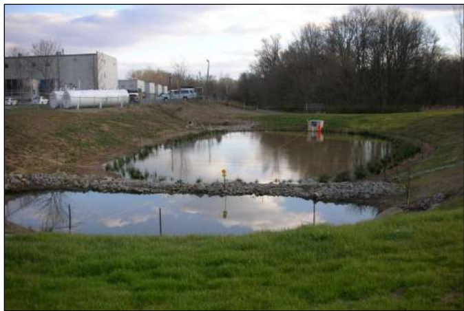
Figure 5.8-2. WDB with Permanent Pool
