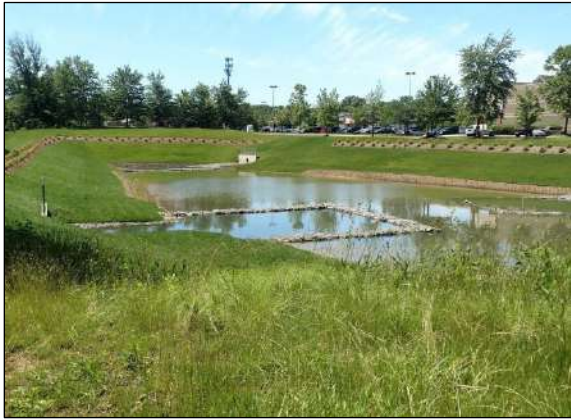
Figure 5.8-1. Wet Detention Basin Source: HDR
