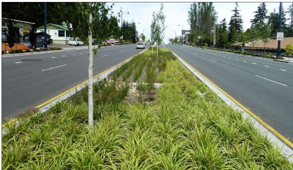
Figure 5.3-3. Bioretention Area within Roadway Median
