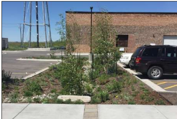
Figure 5.3-1. Bioretention Area Source: Courtesy of the City of Bozeman
