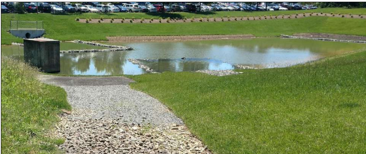
Figure 5.8-6. WDB Maintenance Access
