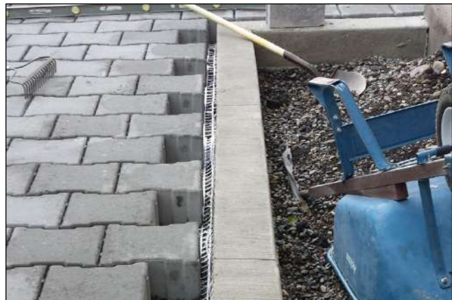
Figure 5.4-7. PICP Installation
