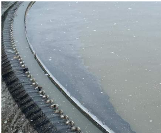
3. Oil sheen seen in Veolia treatment plant pond.
