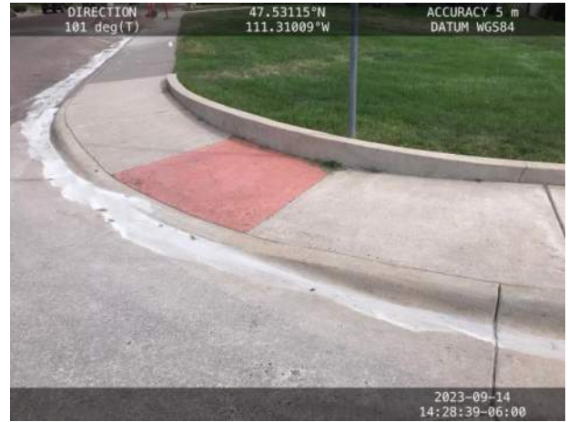
2. Concrete washout flowing along curb line.
