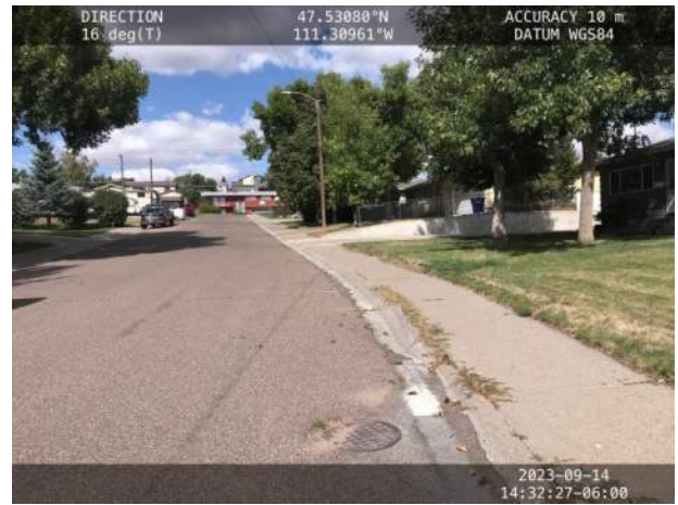
4. Concrete washout stopped flowing in curb line and did not enter storm inlet.
