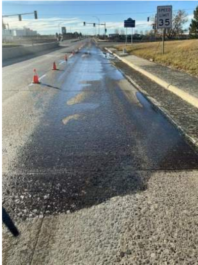
1. Truck with broken fuel tank spilled diesel fuel at intersection of N River Rd and 15 th St NE. Black Eagle Fire blocked off and placed cat litter around inlet.
