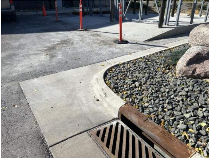
Photo shows concrete washout/cement material from dried ramp work traveling down to the storm inlet
