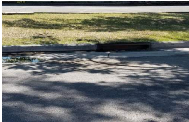
3. Discharged water being pumped from building flows along curb to storm inlet.
