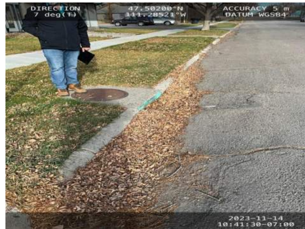
Closest storm inlet can be seen covered with debris and no trace of oil entering MS4. This poses no threat to the MS4.
