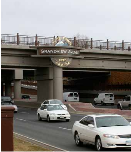
Example of gateway marking element on an underpass
