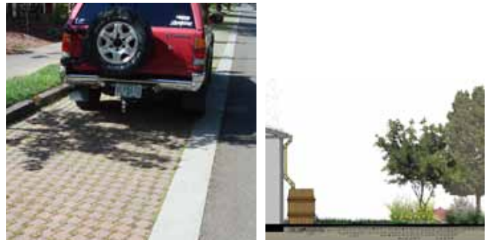
Permeable Pavers in Parking Bays or Roadway and Reclaimed Water for Irrigation System
