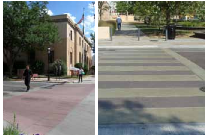
Colored Concrete Crosswalks
