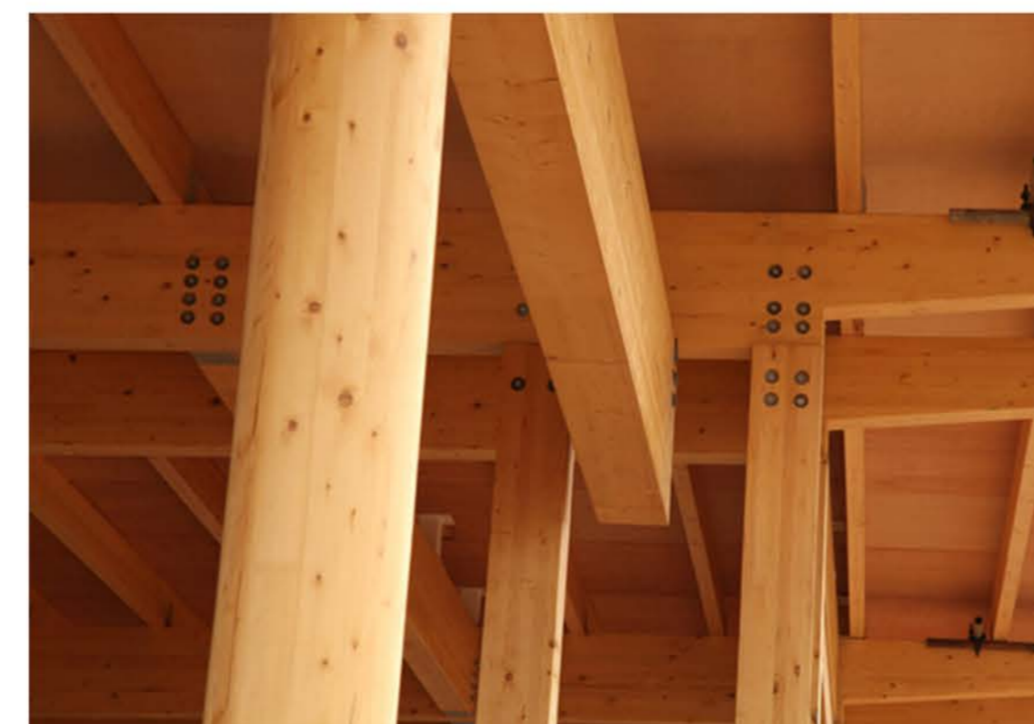
EXPOSED GLULAM BEAMS / COLUMNS WITH BLACK POWDER COATED METAL HARDWARE ACCENTS
