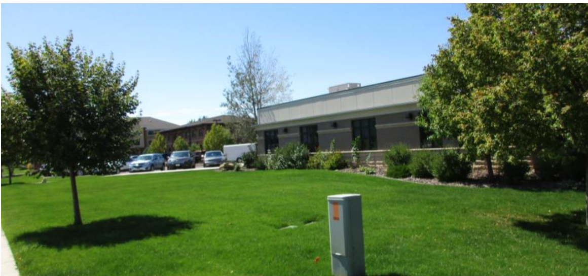
View looking south-west from River Drive South.
