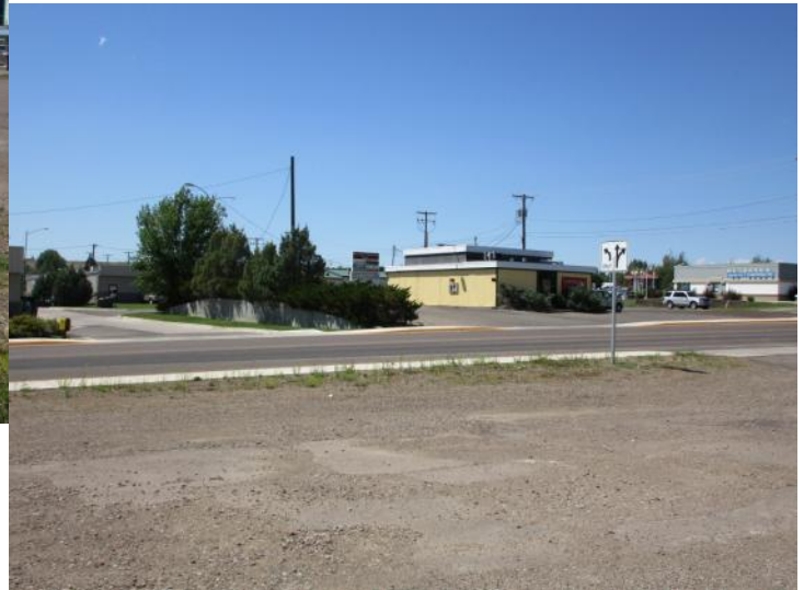
LOOKING NORTHWEST ACROSS SITE SHOWING PROPOSED LOCATION OF CURB CUT ONTO 4TH STREET NORTHWEST; LANE WIDTH NARROWS AT EXISTING CURB CUT
