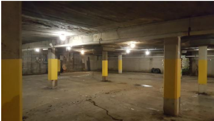
EXISTING CONDITIONS OF THE BASEMENT BELOW SHOWROOM & LOT
