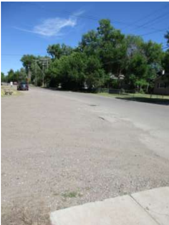
2. Looking east along 10 th Avenue Southwest sidewalk end and gravel extends to public ROW
