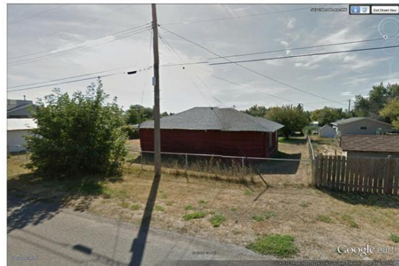
View looking at the detached garage from Colorado Avenue Northwest.
