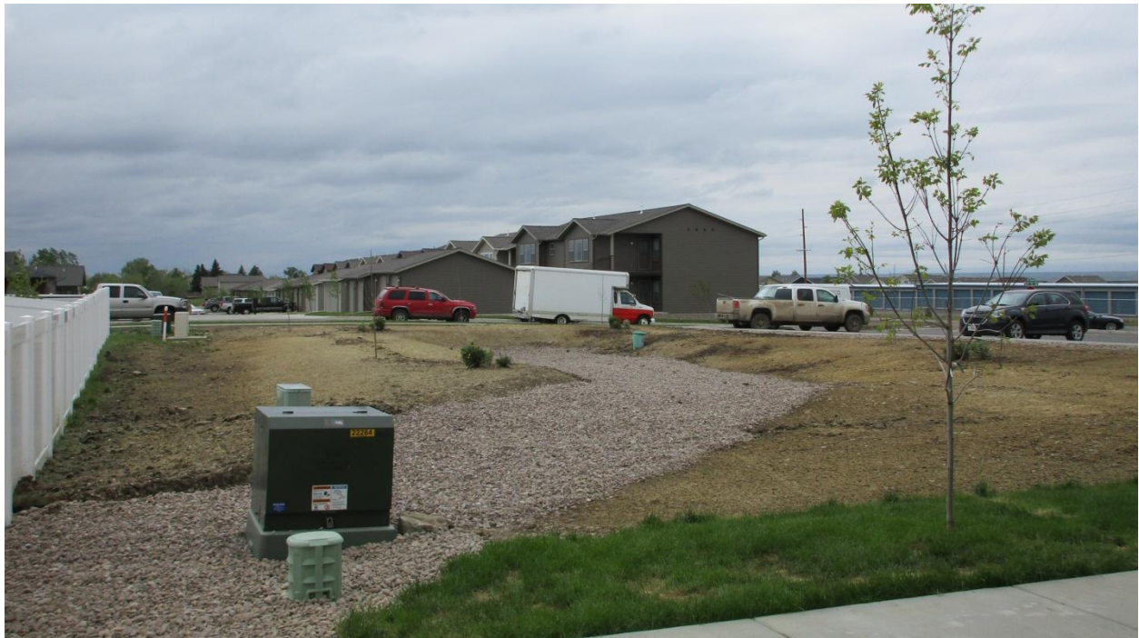
4. Existing Stormwater Basin which will be located on Lot 1A and will be maintained by a shared agreement.
