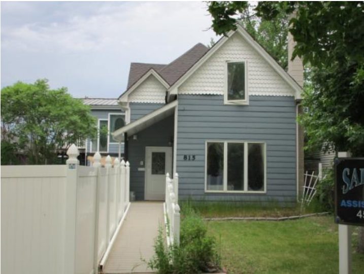
LOOKING NORTH ALONG 2ND AVENUE SOUTH; APPROXIMATE LOCATION OF ENTRANCE RAMP TO REMAIN
