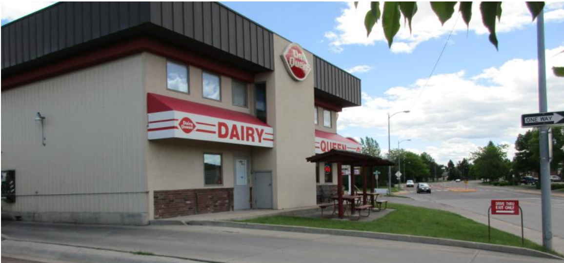
View looking south along Fox Farm Road showing the drive thru lane and the access drive off of Fox Farm Road.
