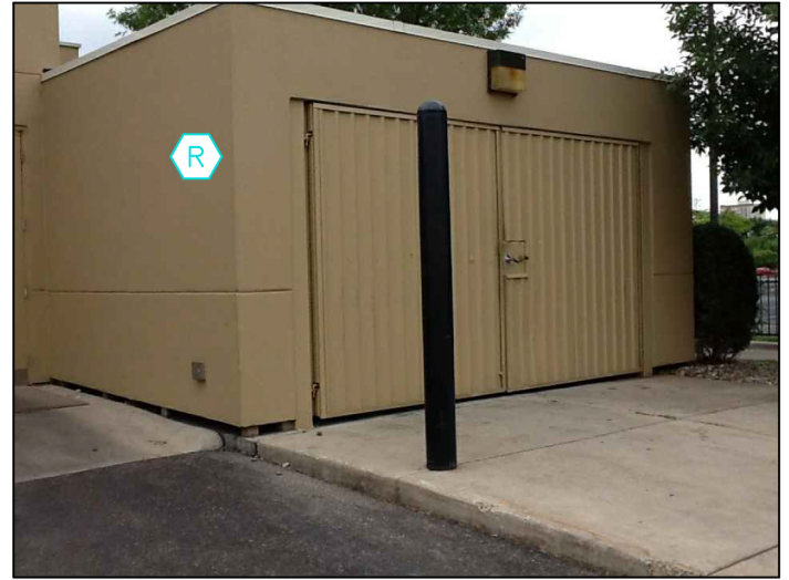
Example of Cooler, Freezer, and Garbage Inclosure. Picture taken at Dairy Queen in Minnesota
