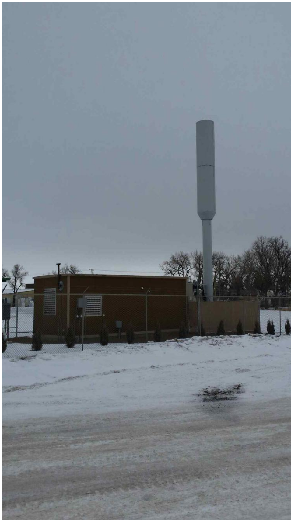
EXISTING 45 FOOT TOWER LOCATED AT 305 6TH STREET SOUTH.
