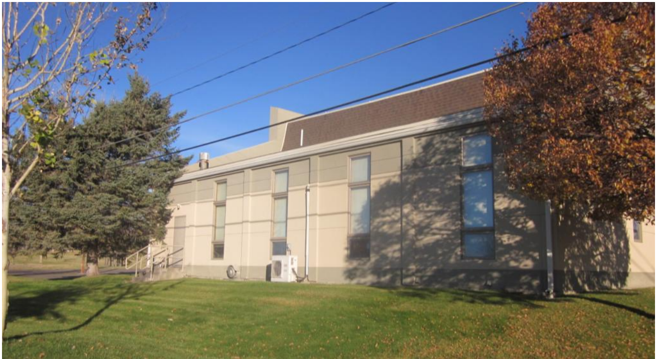
View of existing south elevation.
