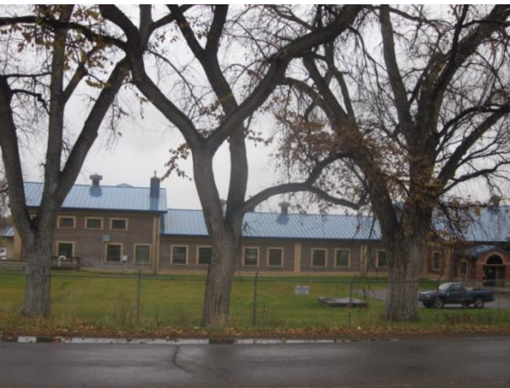
LOOKING NORTHWEST TOWARDS CURRENT FILTER AND CLEARWELL BUILDING FROM UPPER RIVER ROAD; PROPOSED ADDITION TO BE PLACED AT CENTER
