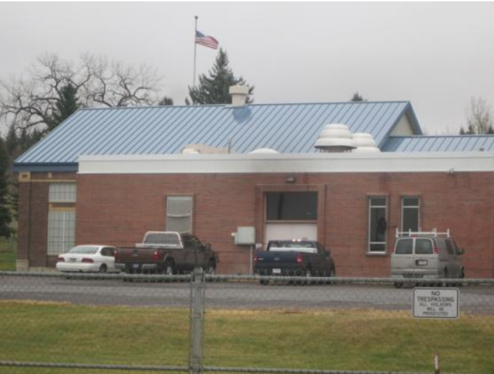
LOOKING EAST TOWARDS CURRENT PUMP STATION AND ADDITION
