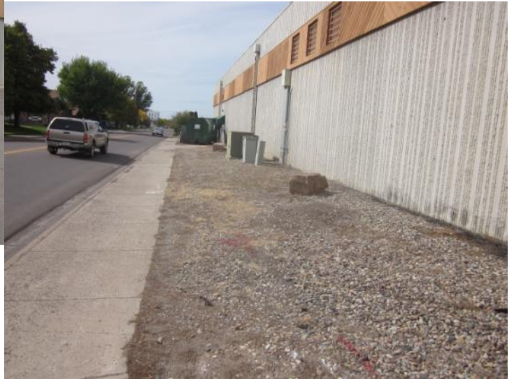
REAR VIEW OF SITE FOLLOWING 11TH AVENUE SOUTH
