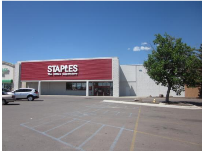
EXISTING FAÇADE OF STAPLES
