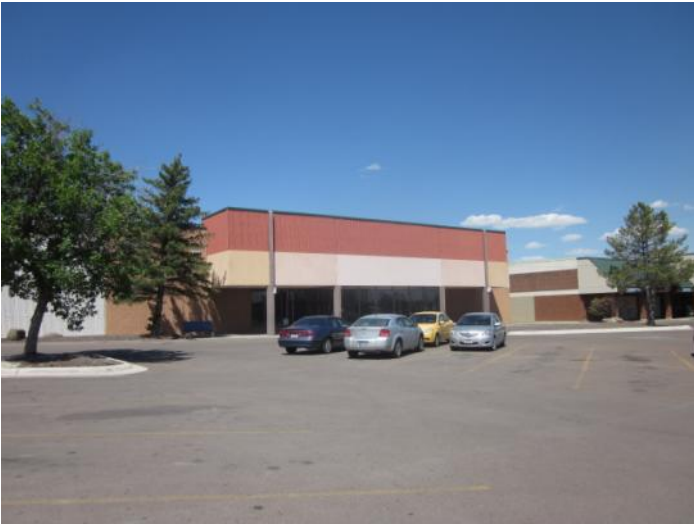
EXISTING FAÇADE OF TJ MAXX
