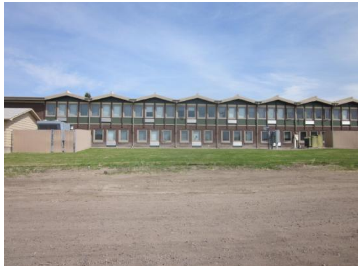
View north from 14th Ave S
