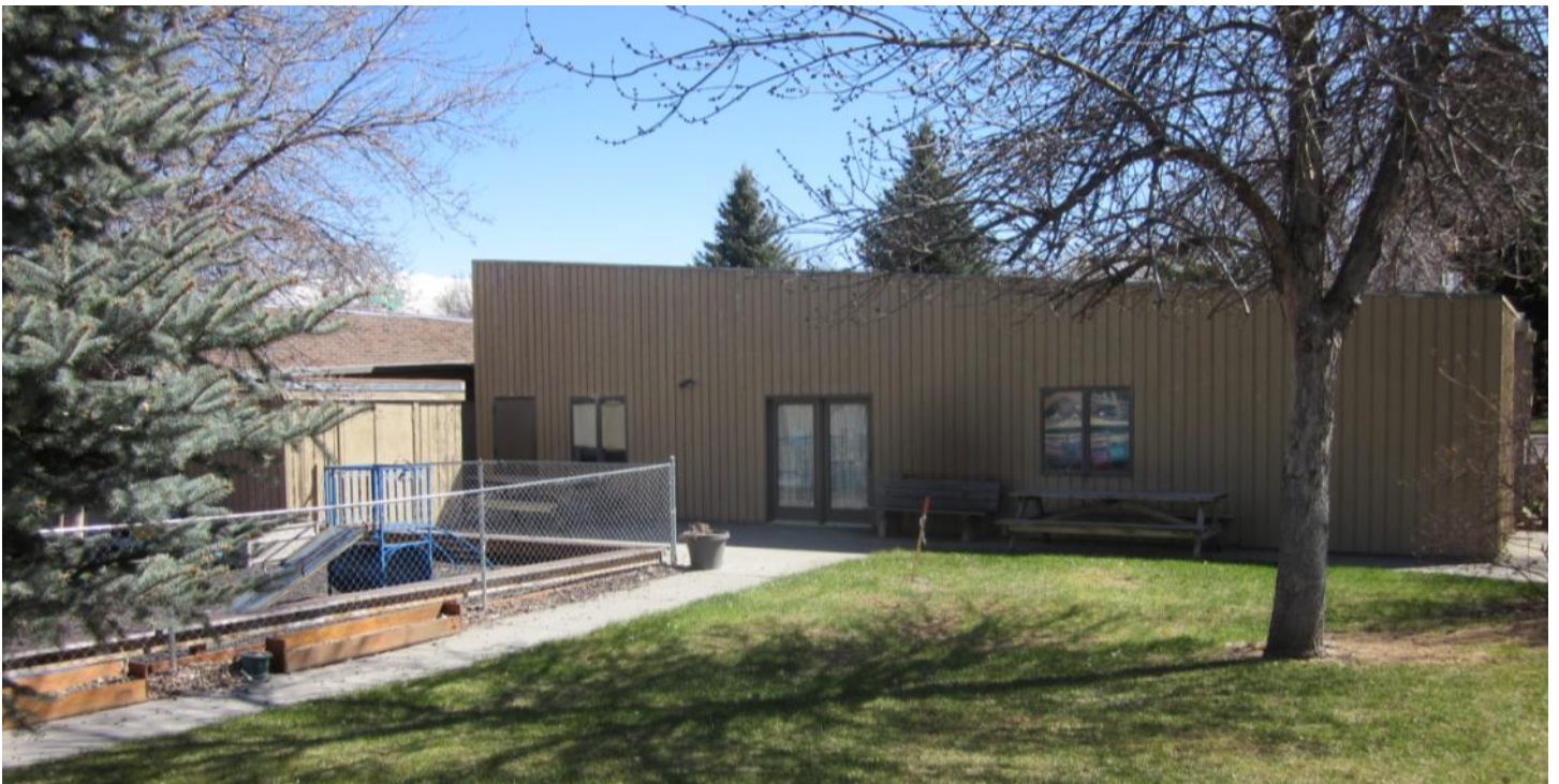
View of existing north elevation.
