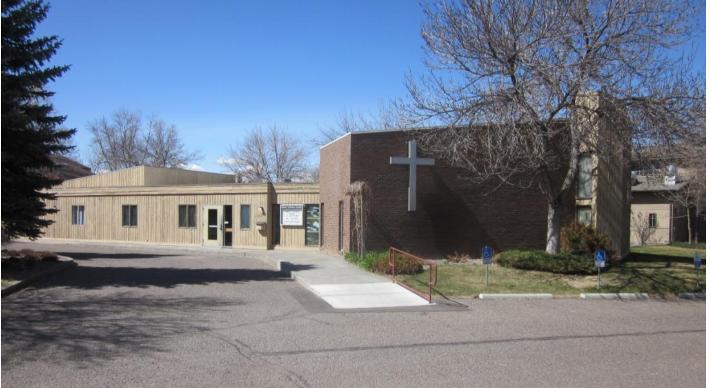
View of existing south elevation.
