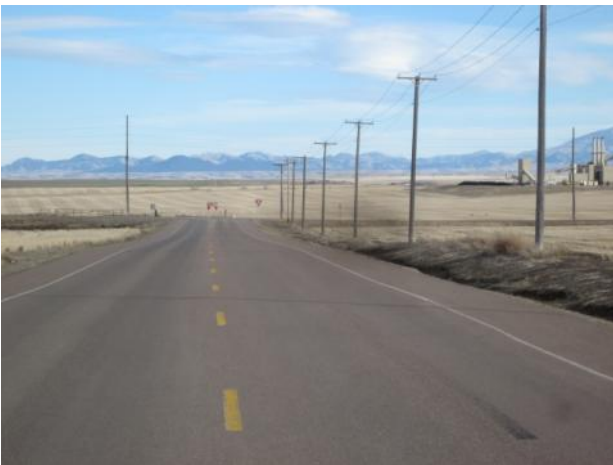
View east along 18th Ave N.
