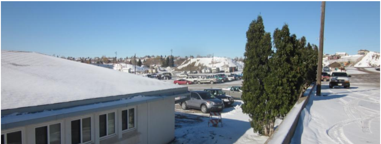
Looking north along the driveway over the proposed project area
