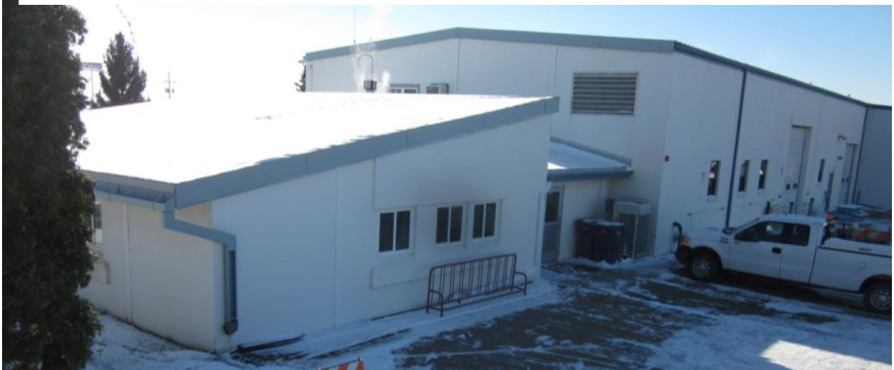
Existing north elevation of the administrative building
