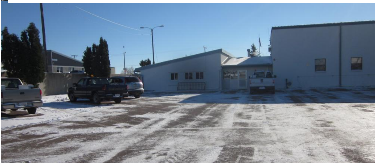
Looking south over the project area
