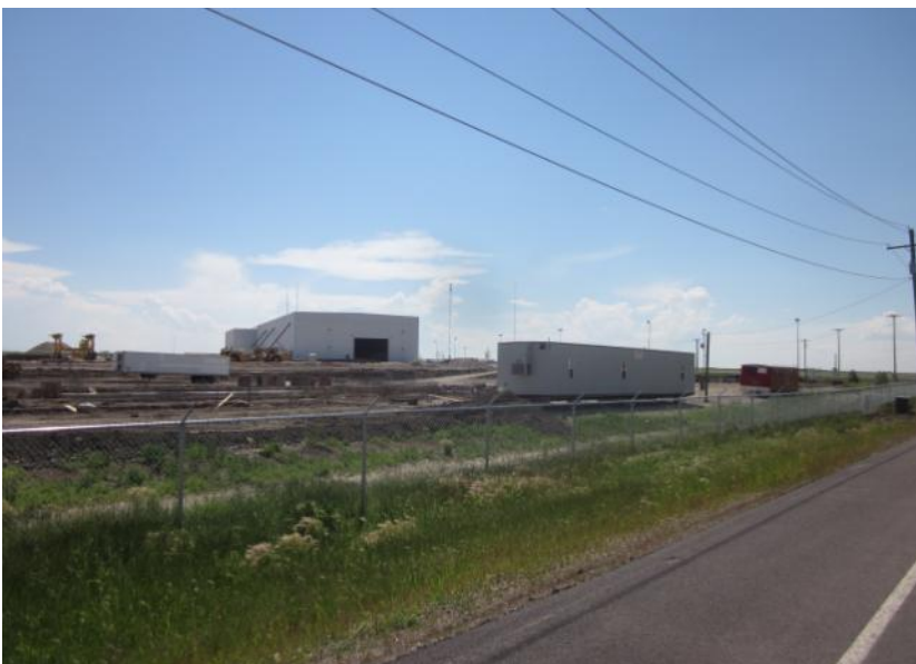
View looking southwest from Great Bear Ave
