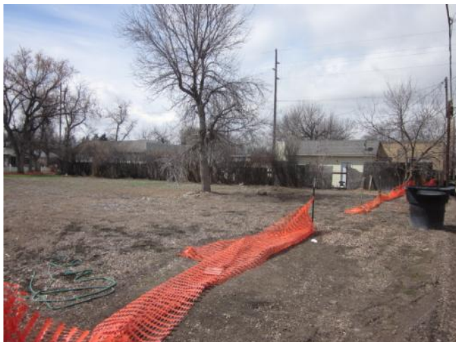
View west down the alley on the north side of Townhomes project site.
