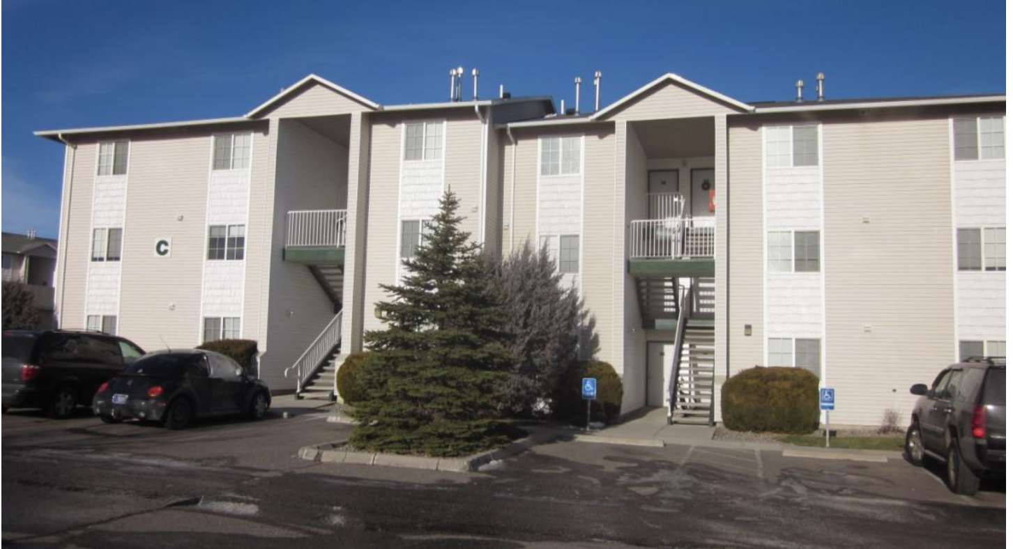
SOUTH ELEVATION OF EXISTING 12 PLEX
