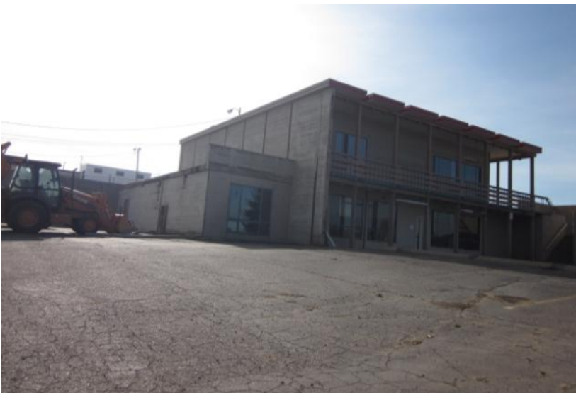
View southeast toward parking and existing building on site
