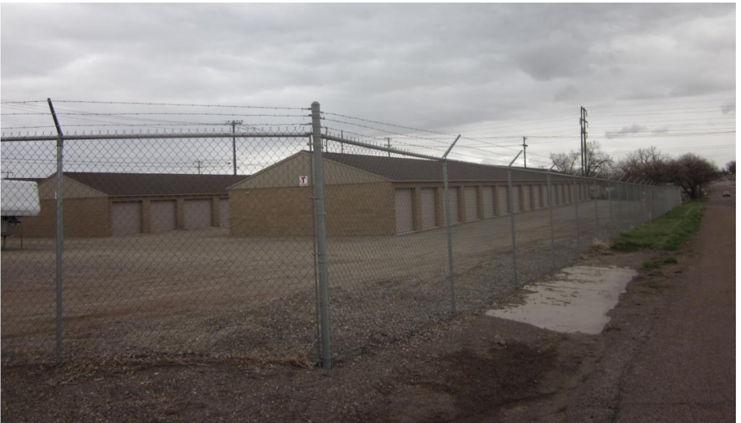
Existing U-Stor-It units and fencing; proposed buildings and fence to match existing
