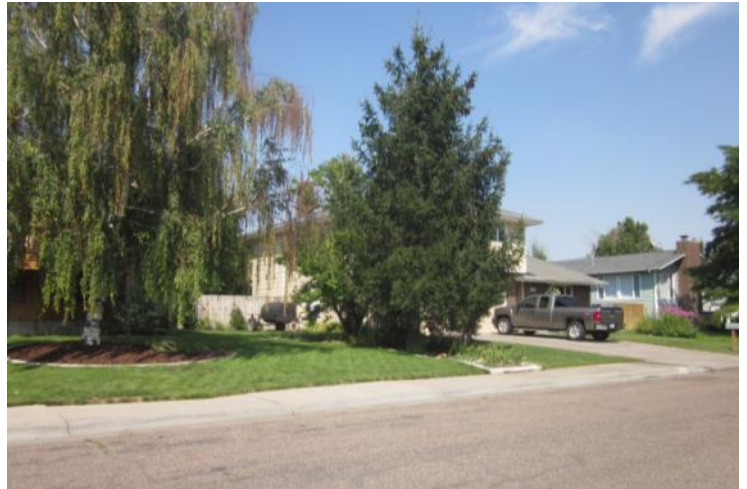
View looking northeast at the location of the proposed garage addition.
