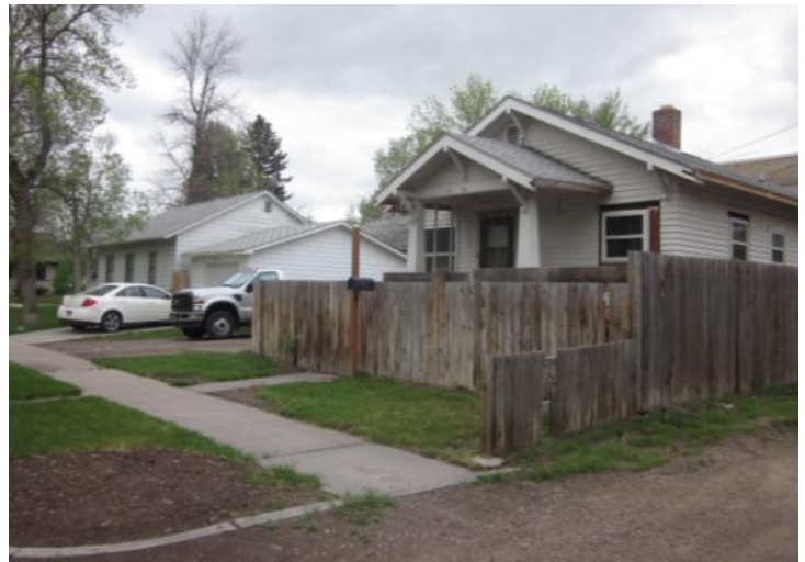
View looking southeast, from the alley, at the subject property in relation to the neighbor to the south who would be most impacted by the proposed garage.
