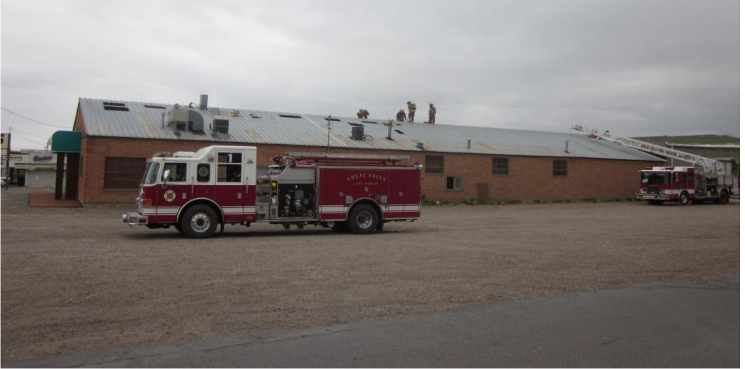
View north of subject property
