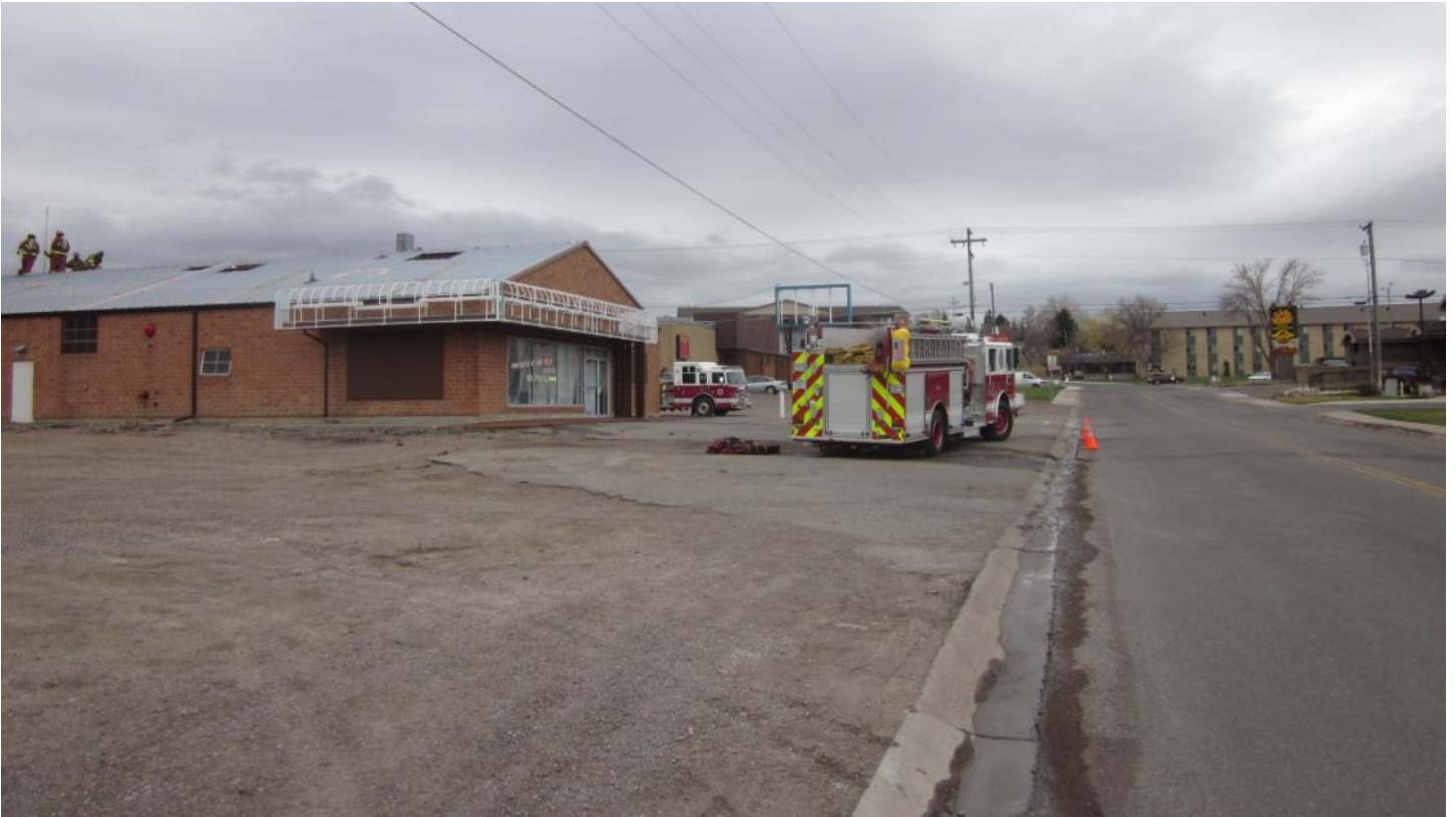
View south down 7th Street South
