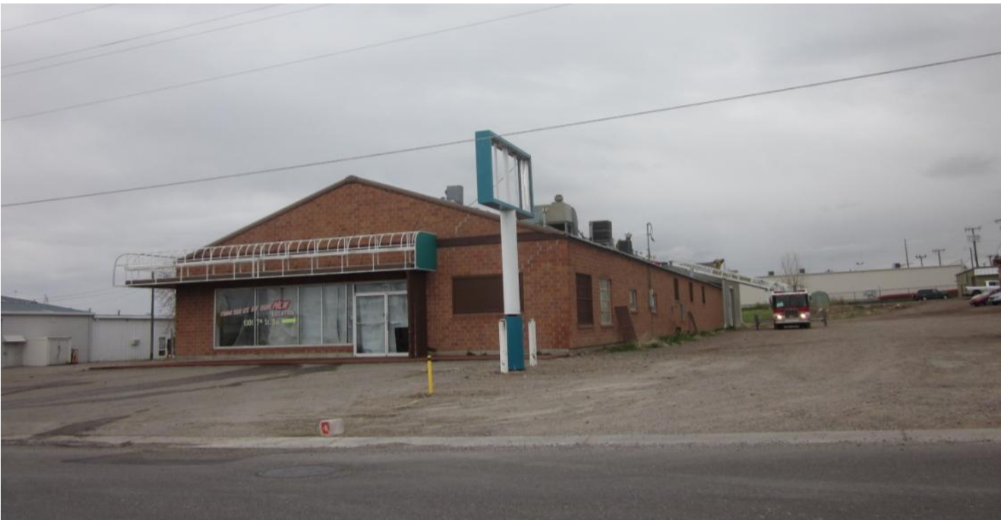
View east from 7th Street South toward existing building on site.
