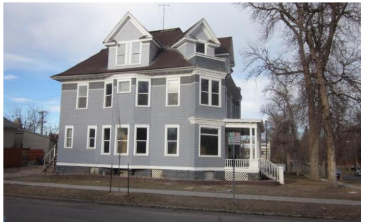
View west from 7th Street North toward existing residence.
