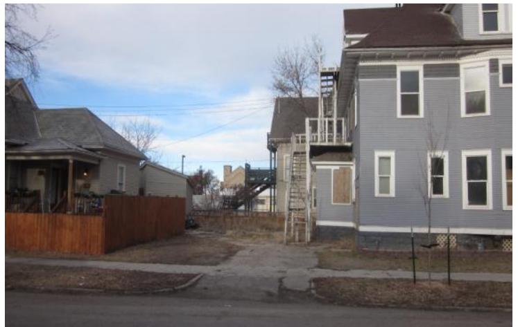
View west toward the back corner of existing residence.
