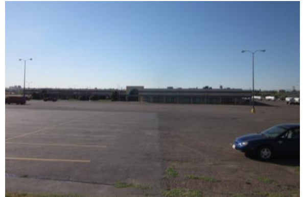
View from 3rd Street Northwest toward Westgate Shopping Center and vacant land to the east.
