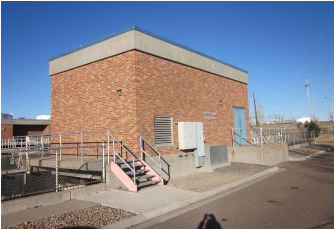
Existing building at Waste Water Treatment Plant; proposed buildings to match.
