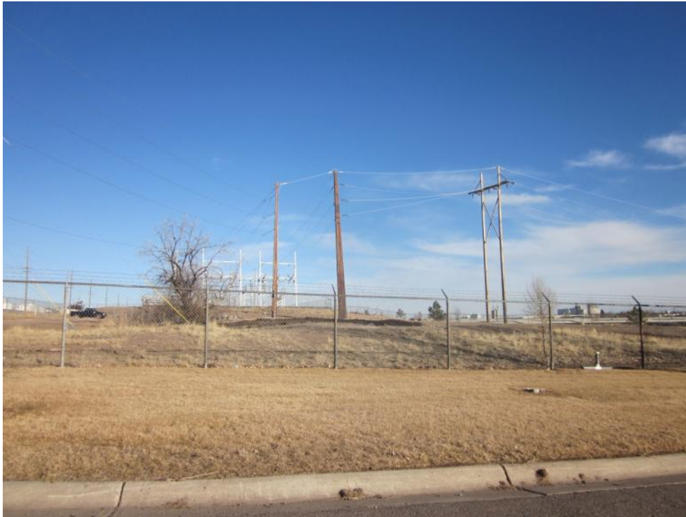
View east toward subject property
