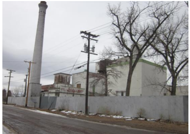
View west down 5th Ave SW, from the southwest corner of the subject property.
