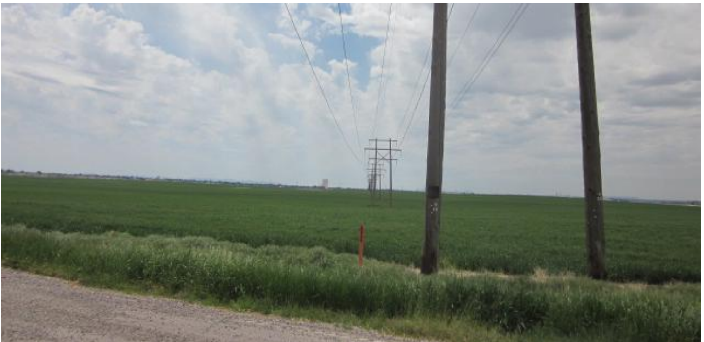
View southwest from 67th St N of subject property and existing utility lines.
