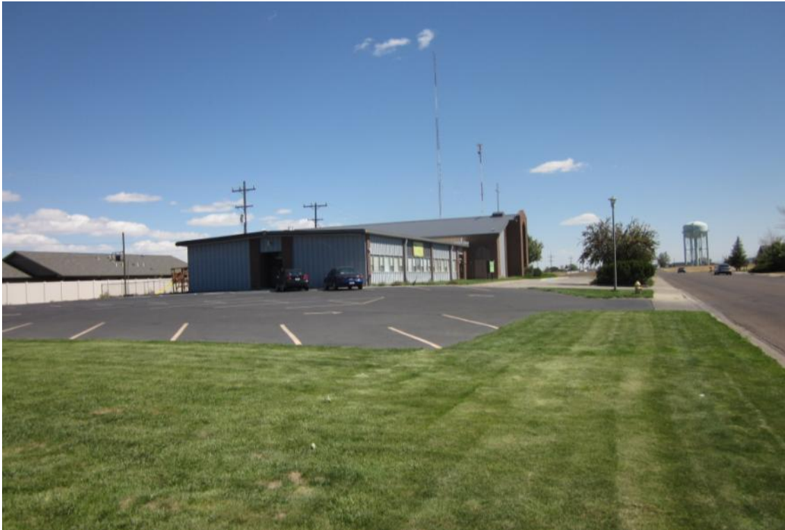
EXISTING PARKING LOT
