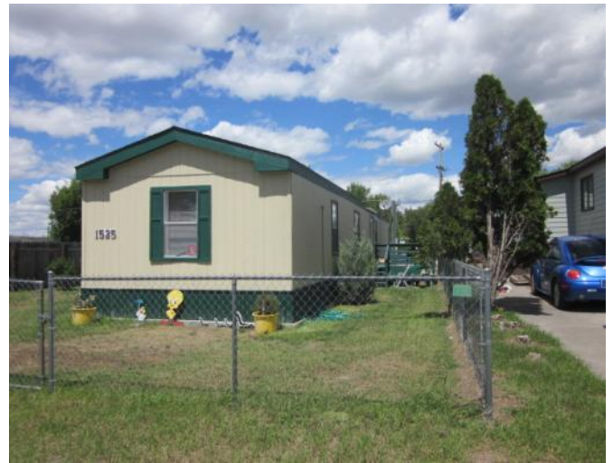
View looking north at the front of the existing structure.
