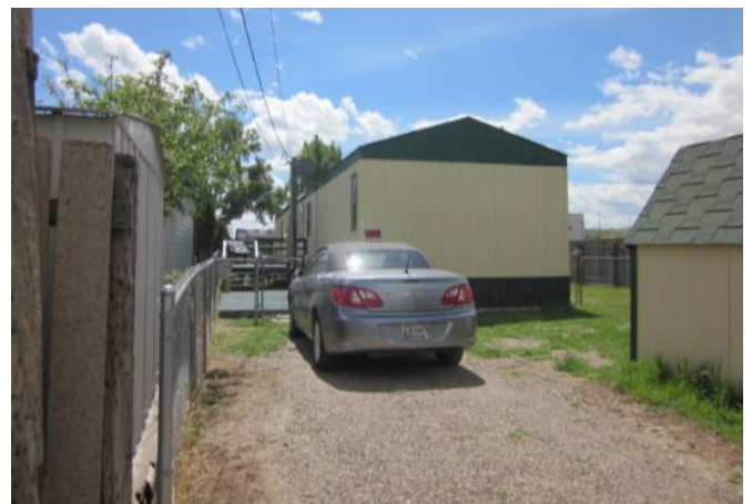
View looking south at the east entry of the existing structure and rear parking area.
