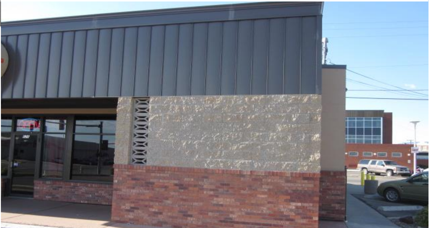
NORTHWEST CORNER OF NORTH ELEVATION
