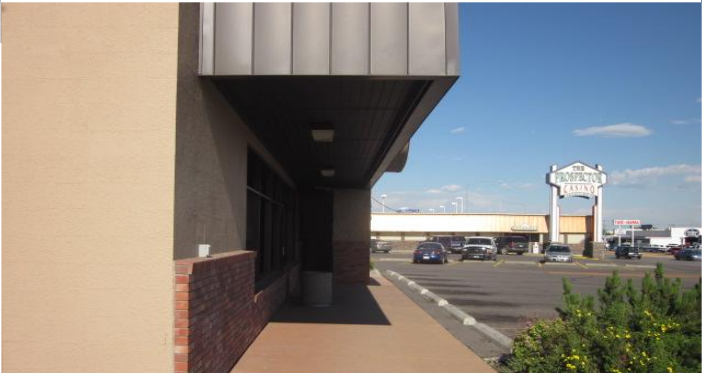
BOX AWNING EXTENDING OVER FAÇADE
