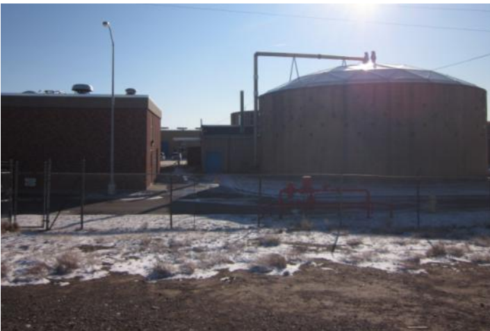
View south toward the City of Great Falls Wastewater Treatment Plant
