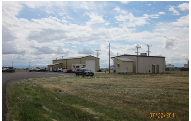
View Southeast toward Lot 1A, Block 1 and washbay.
