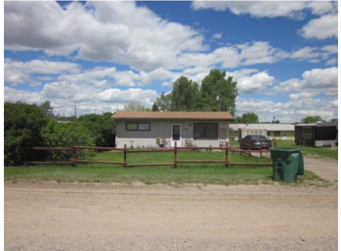
View of residence on subject property.
