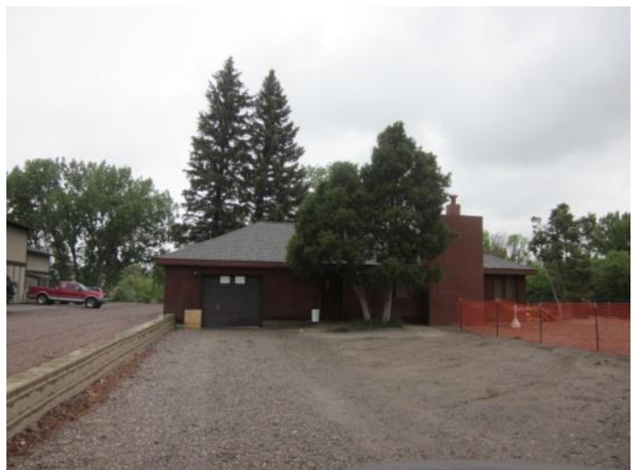
View of residence and driveway on subject property.
