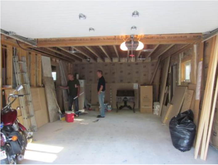
View of Single Stall Garage Area
