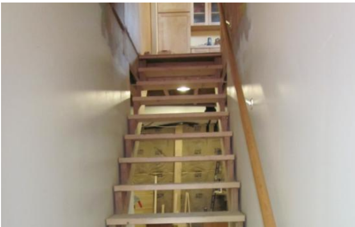
Unfinished Stairs to 2nd Floor
