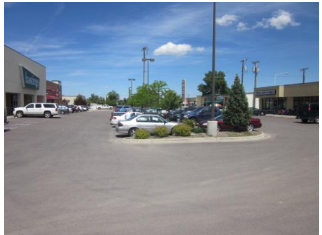
View looking north into the Hastings Parking Lot north of Lot 19A.
