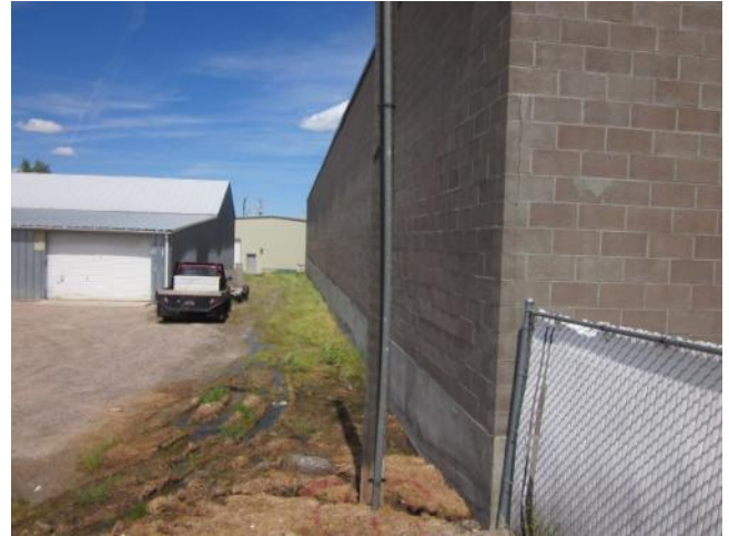
View looking north along the rear property boundary of Lot 19A.
