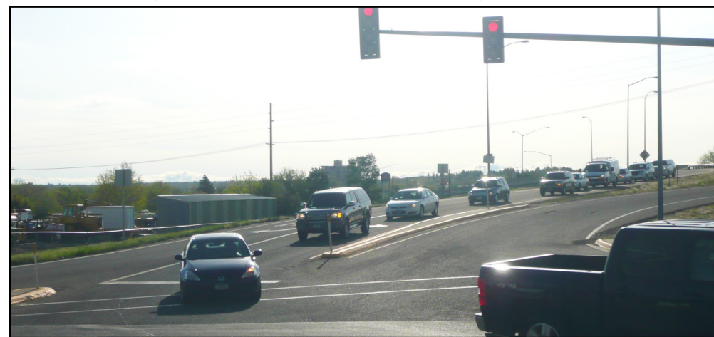
Poor intersection function at the intersection of I-315 Eastbound Off Ramp and 14th St SW can cause vehicle delays on the connecting roadways.
