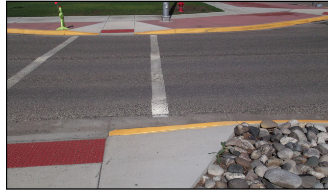
ADA ramps create an easier transition between sidewalks and the streets.
