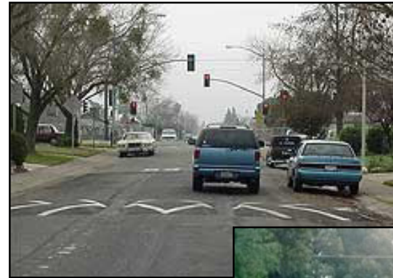
Raised Speed Bumps
