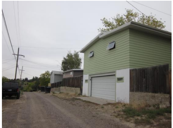
View northwest from alley toward existing garage with proposed second residence above.
