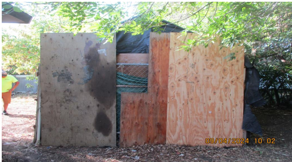
Secured temporary shelter
