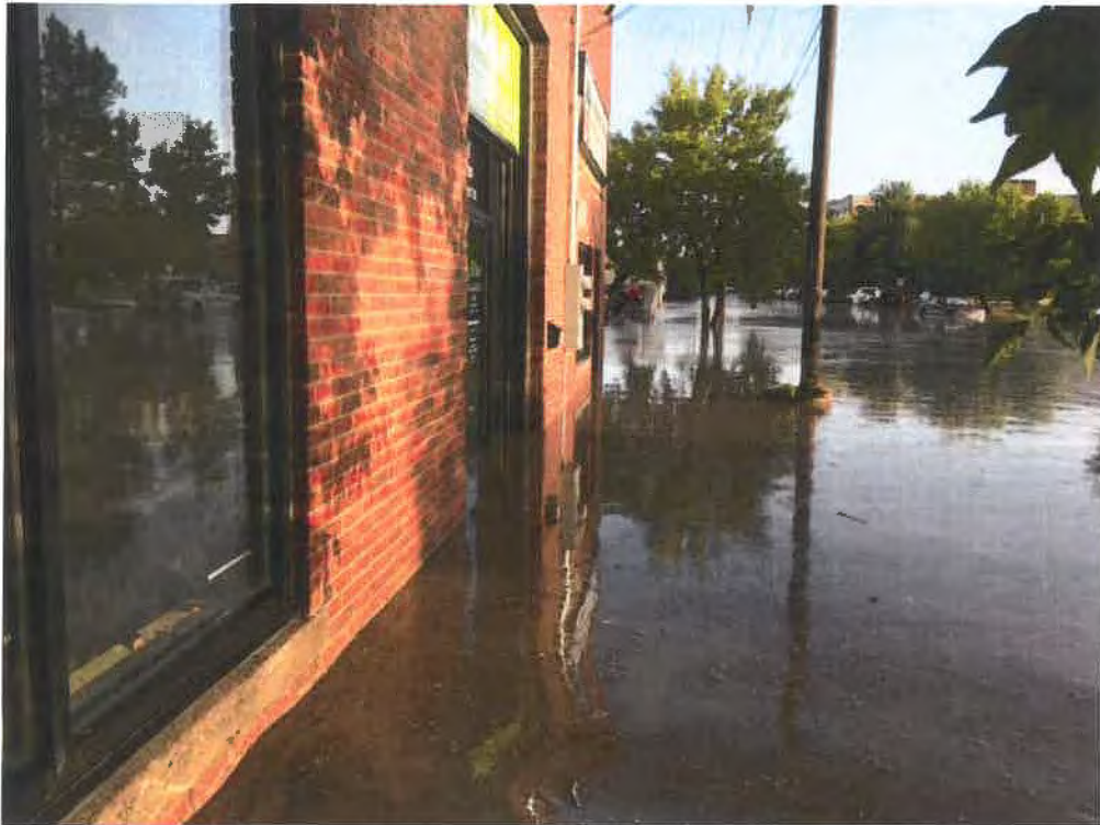
Looking South from Builders Exchange Entry (8-9-16)
