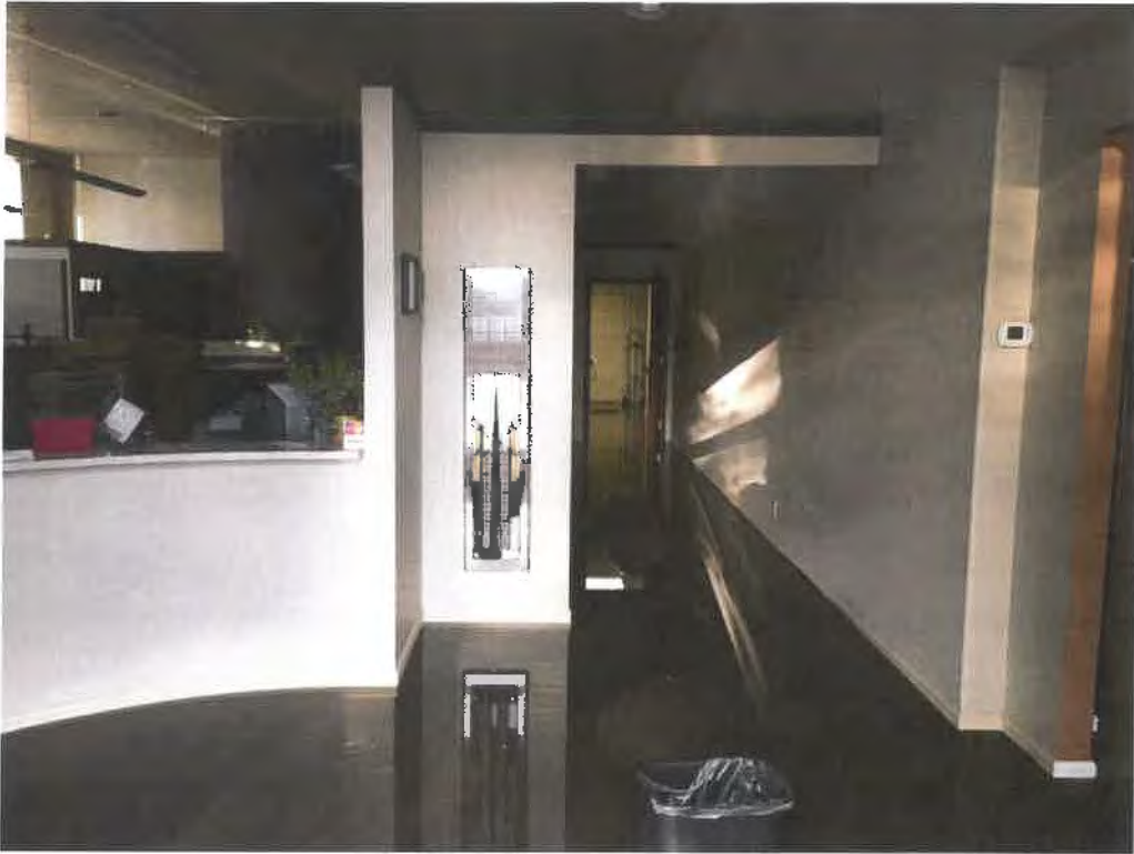
Flooding Inside Builders Exchange (8-9-16)
