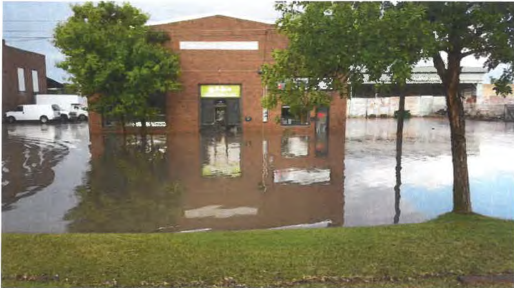
Builders Exchange Flooding (8-9-16)
