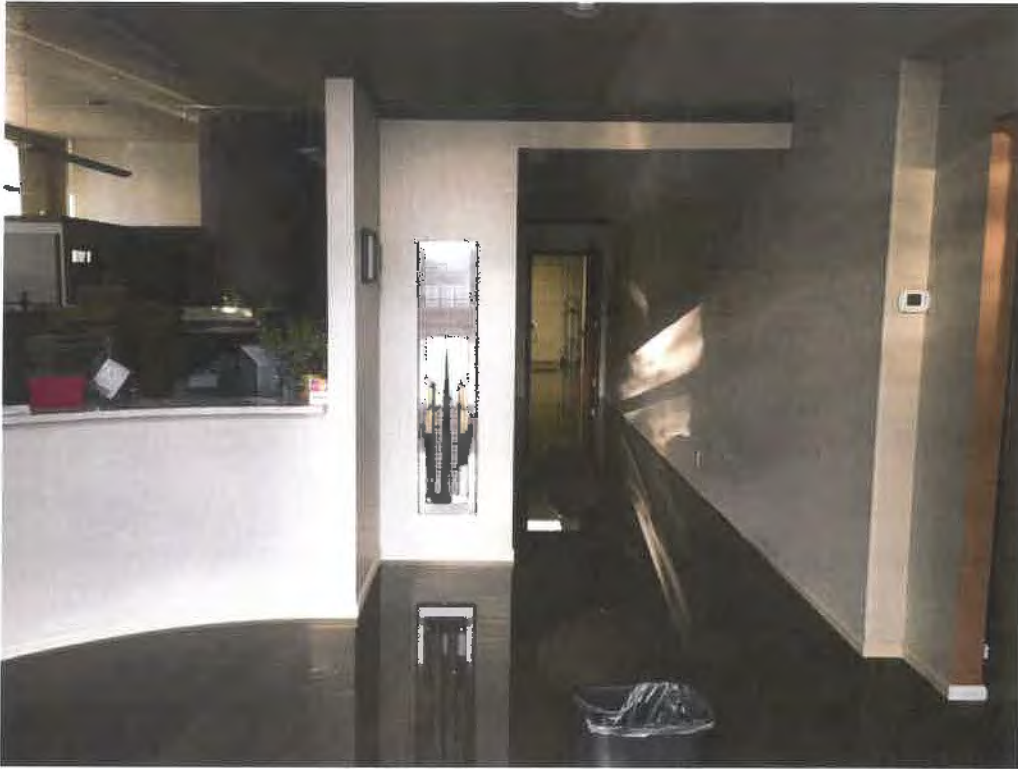
Flooding Inside Builders Exchange (8-9-16)
